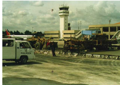
Apron Pavement Works
